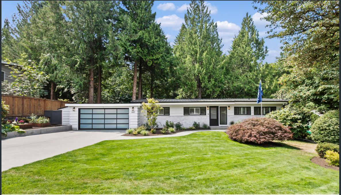
WEST BELLEVUE Full Studs Out Remodel Along a Serene Creek
