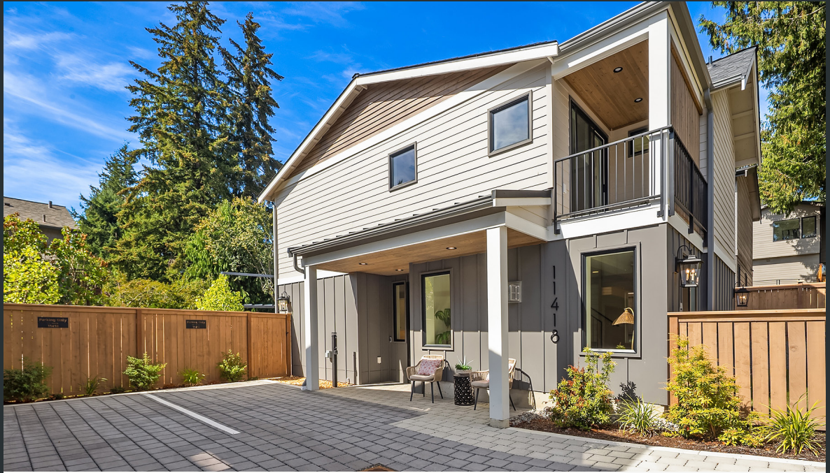
HIGHLANDS Elevated New Construction by Granger & Company
